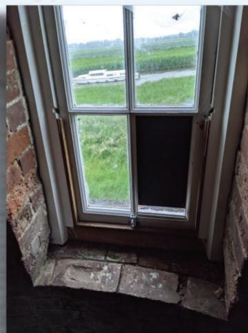
We've been adapting our glazing to incorporate small ledges and gaps for a bat colony to safely enter and leave a mill. We are also leaving gaps around our caps to allow for easy access to the top spaces of the mill.
